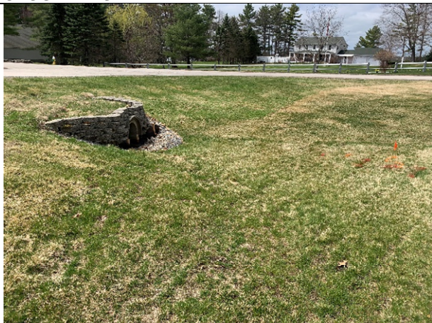
29 Gundalow - 1 (Drainage Area)
