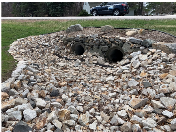
4 Brickyard Circle - 1 (Drainage Course)
